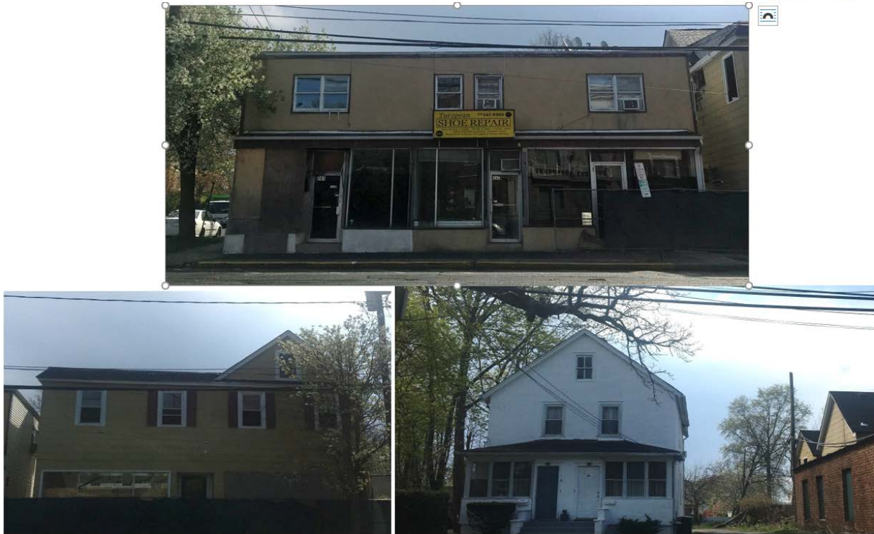
Current Use of the Project Site.
